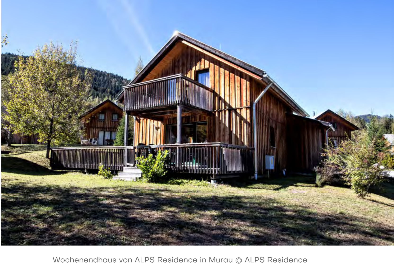
Wochenendhaus von ALPS Residence in Murau © ALPS Residence
